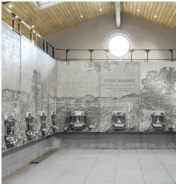
14 Tailor made Standard tanks custom embedded for Château Beauséjour Duffau Lagarrosse in Saint Etmillion
