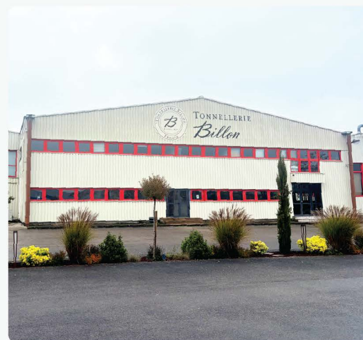
Renovated Billon cooperage facade.
