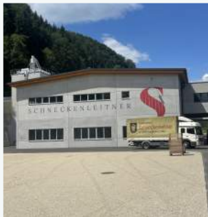
New Schneckenleitner cooperage completed in 2022.
