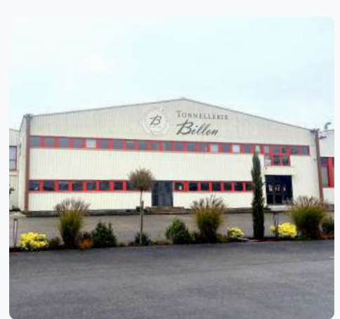
Renovated Billon cooperage facade.
