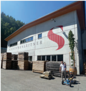
The new facade of the cooperage and Paul Schneckenleitner with his sons.
