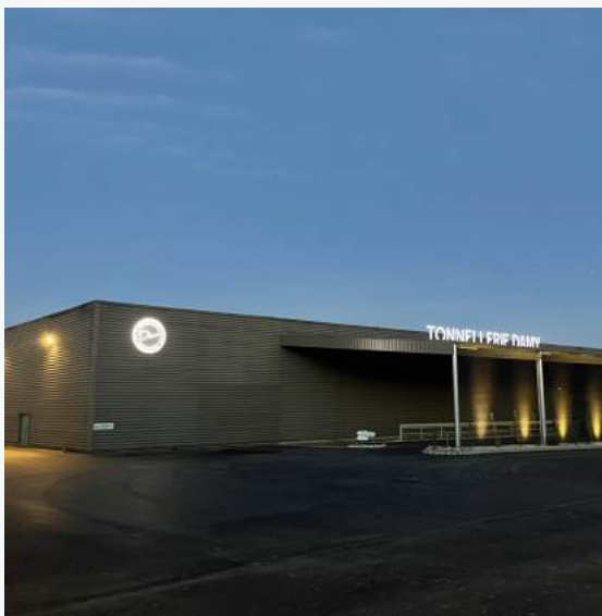
New loading dock covering with incorporating solar panels and future green wall.
