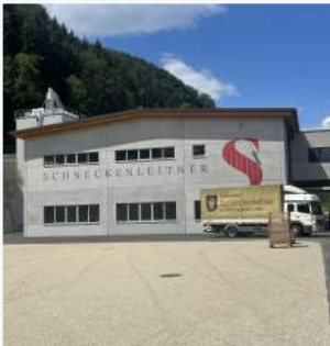
New Schneckenleitner cooperage completed in 2022.
