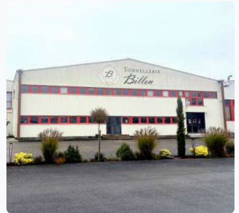
Renovated Billon cooperage facade.
